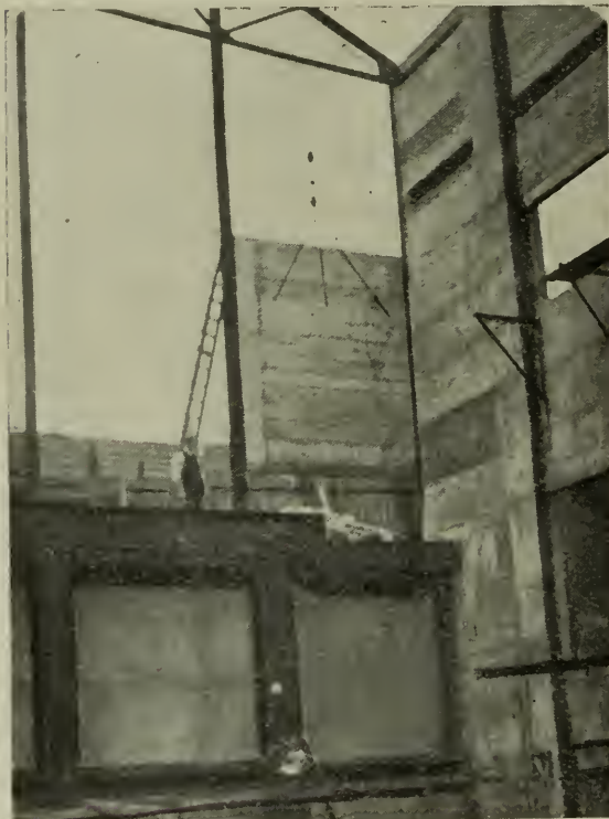
FIG. 2. CONCRETE SLAB BEING LOWERED INTO POSITION.
